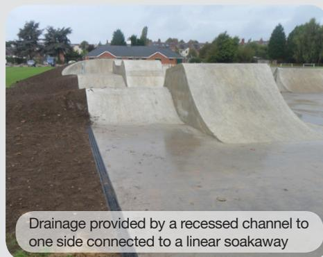
Drainage provided by a recessed channel to one side connected to a linear soakaway
