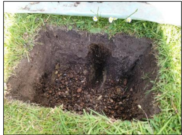
Figure 12. Excavation of slit drain – TP1.
