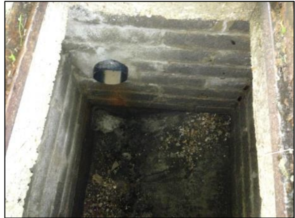
Figure 6. 150 mm carrier drain connected to IC 1.
