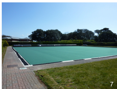
Shockpad installed awaiting installation of carpet (and rubber sheet to be laid into ditches)
