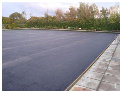
Macadam base after checking before carpet installation
