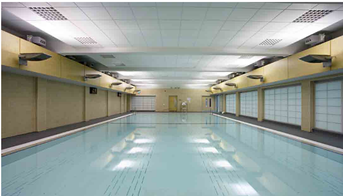
Example of pool with wall mounted luminaires
